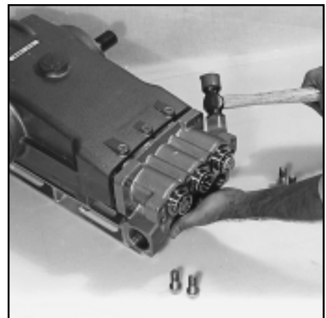
Removing the Inlet Manifold
